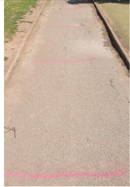
Markers on floor outside to show safe distances
